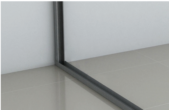
Step 3: Install C studs vertically along wall ends. Fasten studs to wall using applicable fasteners spaced at 100mm (maximum); rest at 500mm (maximum).
