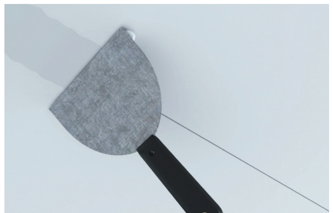
Step 8: Use USG Boral Premium Jointing and Premium Premix and paper tape to have a complete jointing system.
