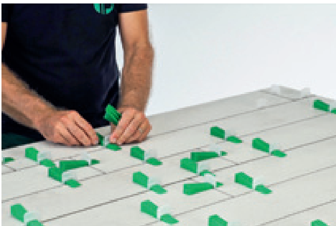
levelling wedges insertion
