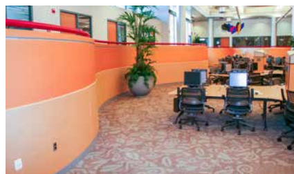
Wainscoting on Curved Stem Wall for Wall-Protection & Acoustics
